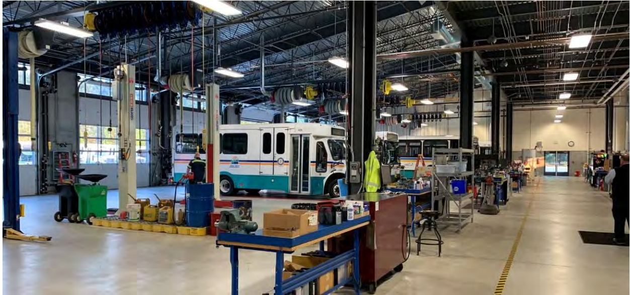
Figure 4 Whidbey Island Facility Maintenance Building Interior
