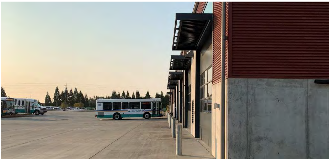
Figure 3 Whidbey Island Facility Maintenance Building and Outdoor Vehicle Storage
