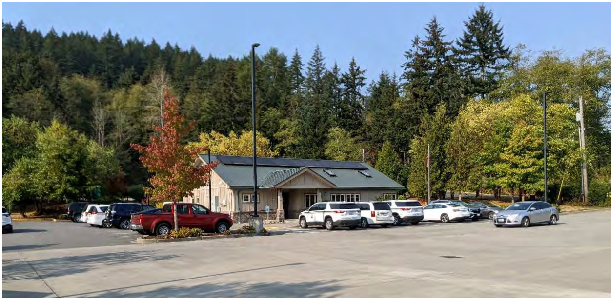
Figure 5 Camano Island Facility
